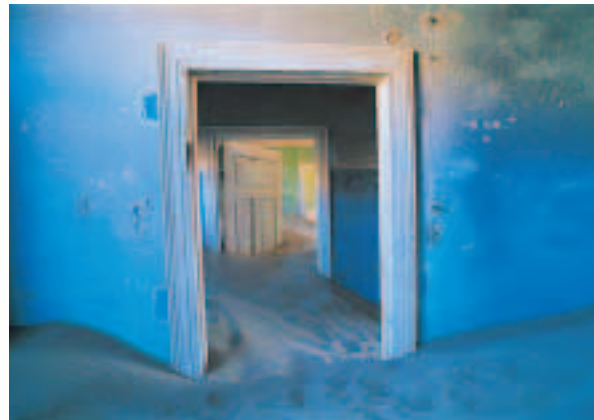
Sand overwhelms building, Namibia
