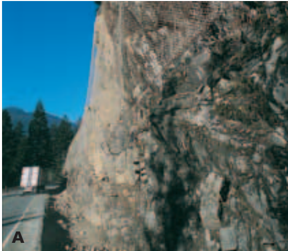
Figure 8-10 This steel net was installed along Route 101 near Quilcene, Washington, to protect motorists from rockslides (A) . In Wolf Creek Pass, Colorado, a fence was built along this highway to protect motorists from rock slides (B) .
