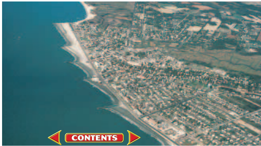
Figure 7-15 Groins at Cape May, New Jersey, are used to protect the beaches from wave erosion. Groins are vertical walls of rock placed perpendicular to the shore to trap sand from ocean currents.
