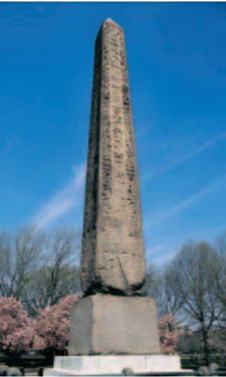
Figure 7-1 This 3600-year-old monument, Cleopatra's Needle was moved from Egypt to Central Park, New York City. After many years in New York City's climate, some markings on the monument have all but disappeared as a result of weathering.
